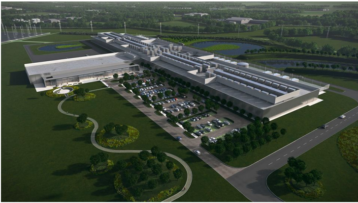
Facebook Datacenter, Clonee, Ireland
